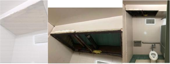
The recent rains revealed failing moisture seals under the CHS stadium bleachers causing significant flooding in the ceiling of a bathroom in the breezeway. Maintenance team members responded quickly to mitigate additional damage.
