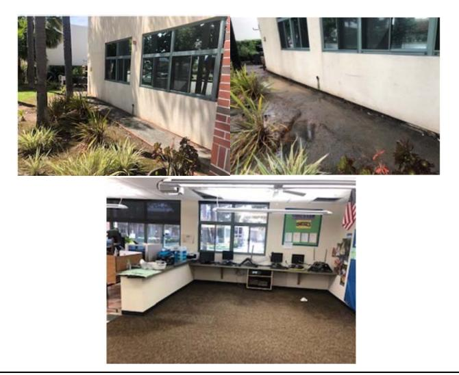
**Above:** The recent rains caused flooding in CHS Building room 701. A well-intended volunteer project resulted in the diversion of water above building flashing that is designed to keep moisture out. Earlier this year, the M&O department implemented the use of a "site improvement form" to provide an oversight and approval process that will ensure adequate review of any changes in our school facilities.
